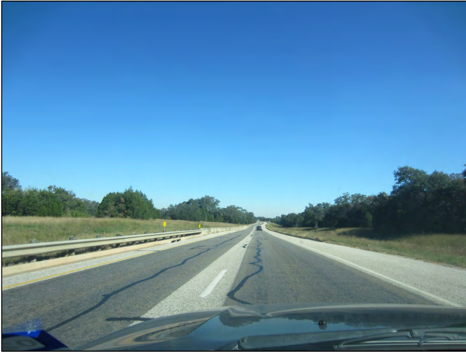
Figure 2: Looking southeast at intersection of MoPac and LaCrosse Ave from southbound MoPac.
