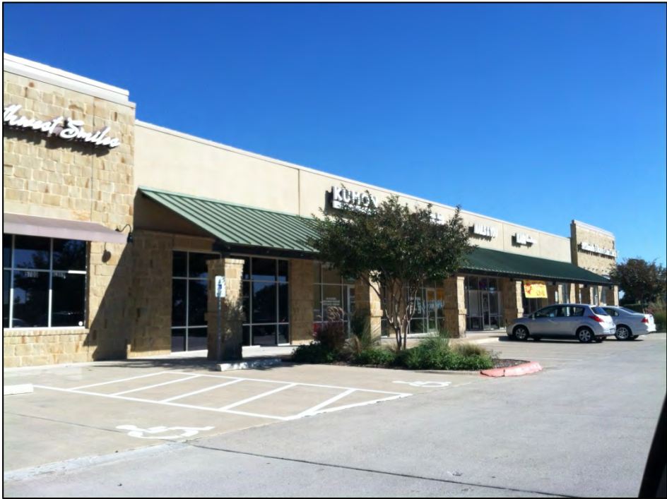
Figure 3: Representative commercial buildings along northbound MoPac at Slaughter.
